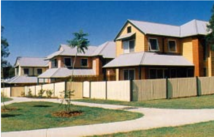
Figure 5: Integrated public housing project, Enoggera, Brisbane
